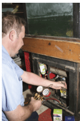
Steve applies Dry-R to the lobster tank.
